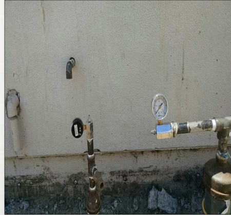
Storm drain tie in and gas line pressure testing
