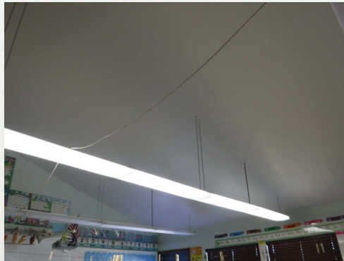
Replaced damaged sheet rock and paint caused by six-year old roof leak
