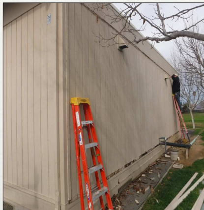
Replacing Rotted Siding on portables throughout the District
